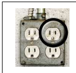
One outlet shown circled.
